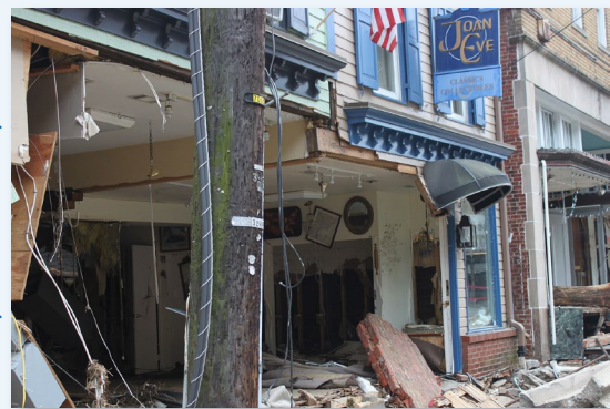
Buildings damaged by one of two "thousand-year" floods to hit Ellicott City, MD since the summer of 2016.
